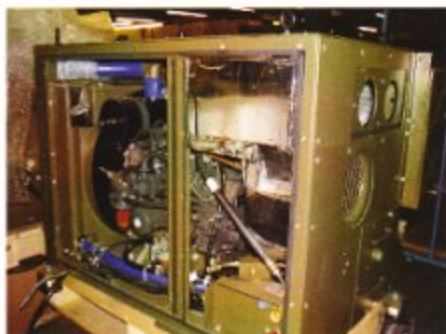
Access Panel Removed
